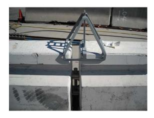
Place the pin puller on top of the pin.
